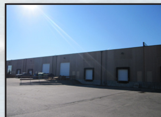
Loading Area with Doors
